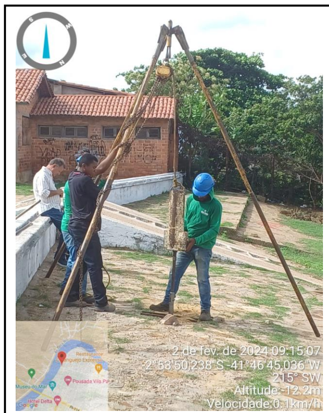
Foto 01: Realizando as Sondagens.
