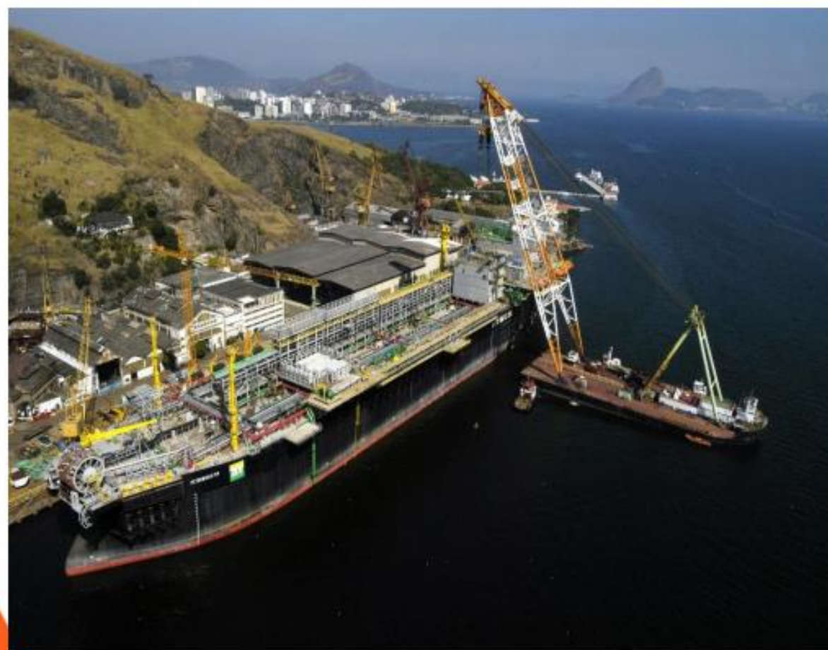
Module integration by Floating Crane Pelicano 1 on FPSO P-54
