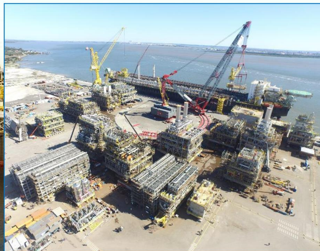
Mechanical Completion of topside modules and starting of the lifting campaign at EBR
