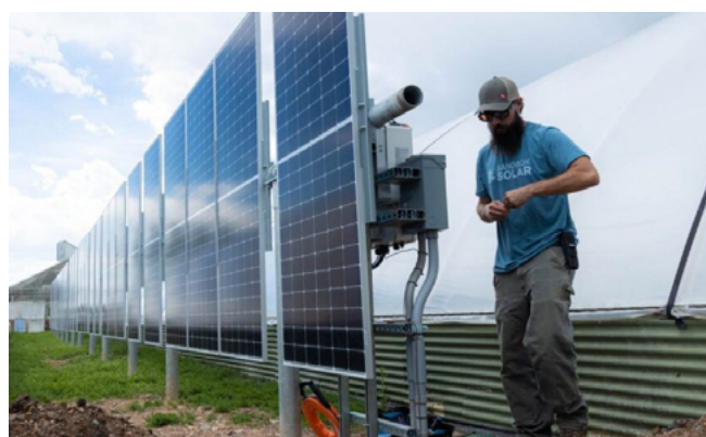
Figure 8 - Vertical photovoltaic system associated with greenhouses
