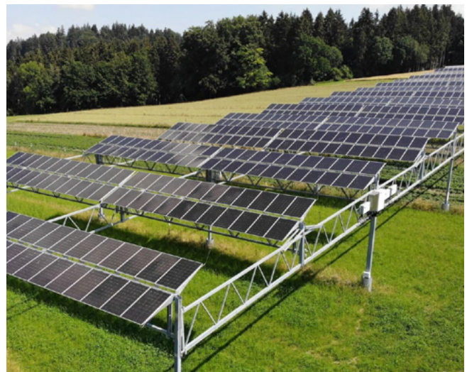
Figure 14 - Heggelbach project built in 2016
