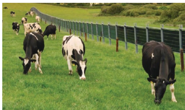
Figure 7 - Bifacial PV modules used as livestock fencing
