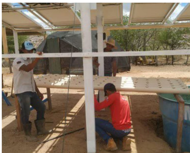
Figure 33 - Agrivoltaic system and assembly of aquaponics system below the modules
