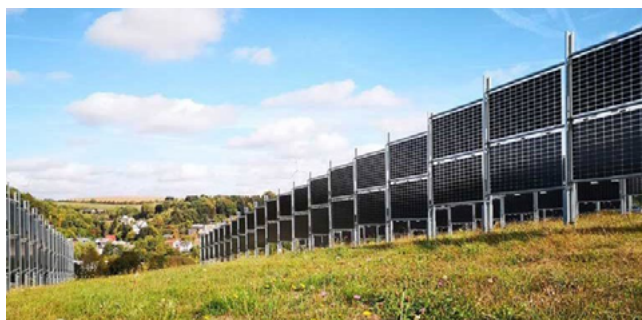
Figure 64 – Bifacial, vertically installed PV modules for fencing applications
