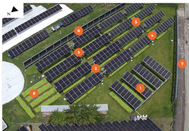
Figure 41 – Aerial view of the Fotovoltaica/UFSC and Repsol agrivoltaic system
