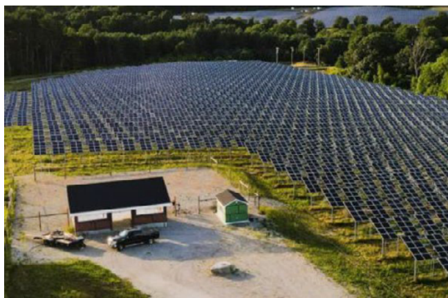
Figure 25 - Grafton Solar agrivoltaic project
