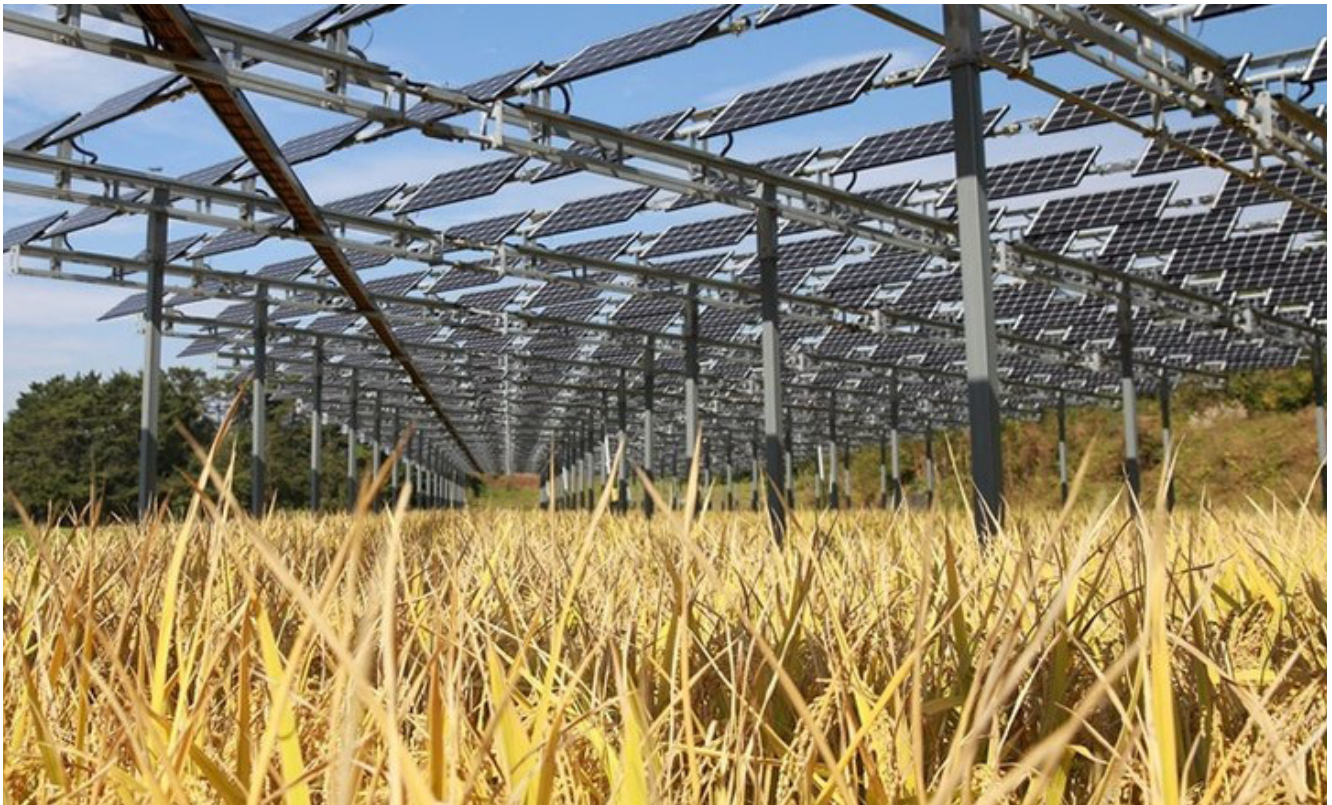
Figure 26 - Agricultural PV system developed by Q CELLS on farmland in Gwandang Village, Namhae
