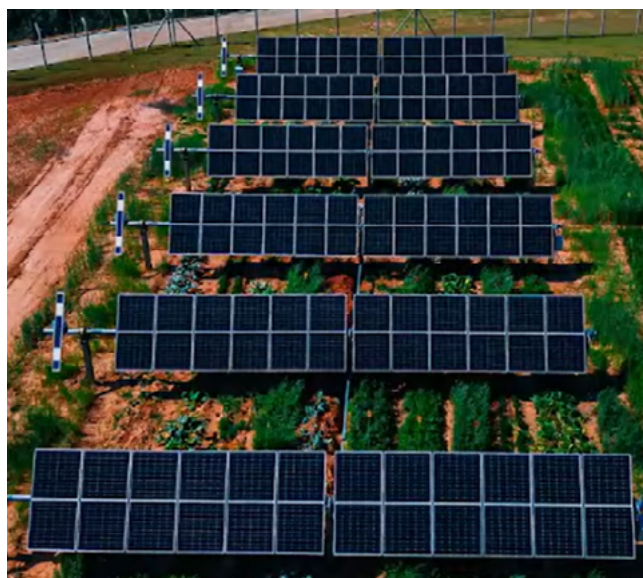
Figure 39 – One of the pilot systems at the Agri Solar Farm
