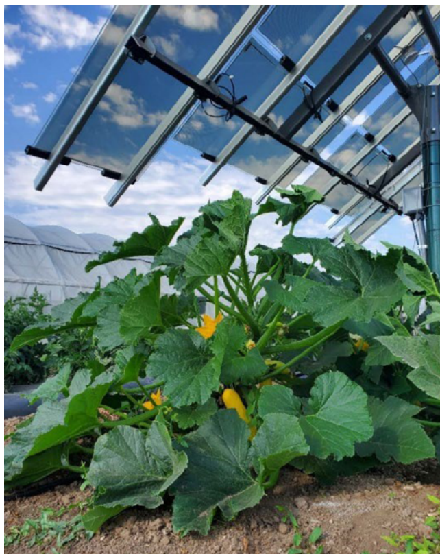
Figure 9 - Agrivoltaic research site featuring monofacial, translucent, and bifacial PV modules
