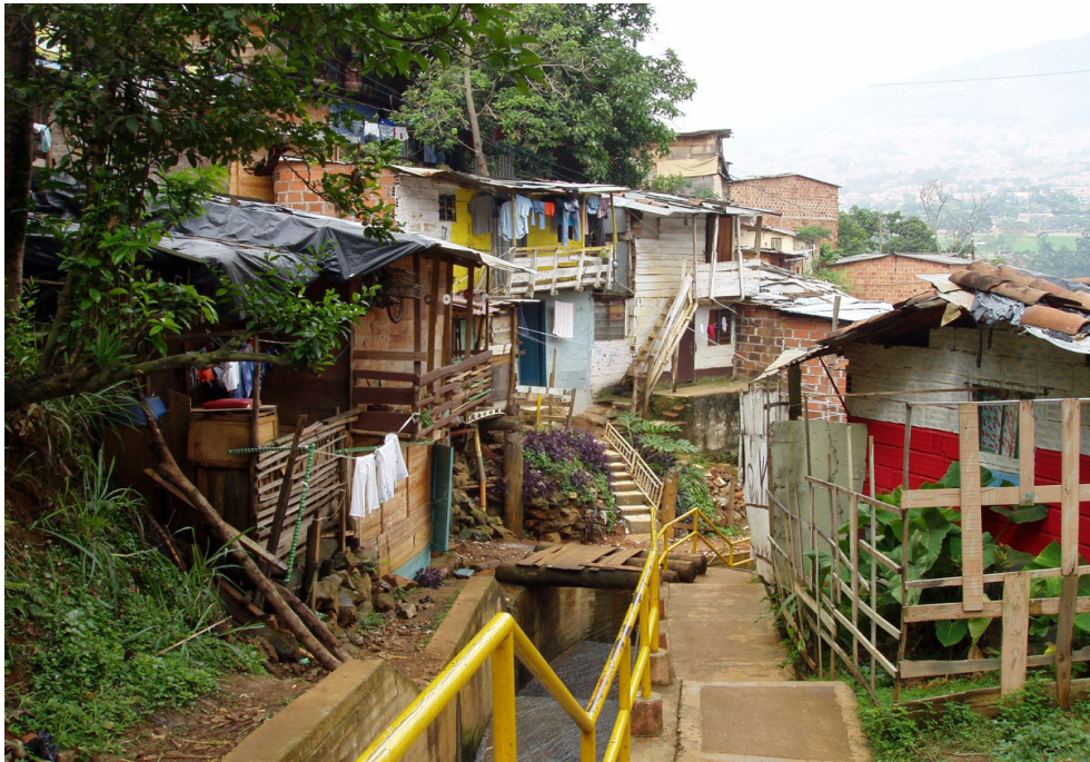
Figure 17. Situation before the intervention in the Juan Bobo stream. Source: EDU, 2004.
