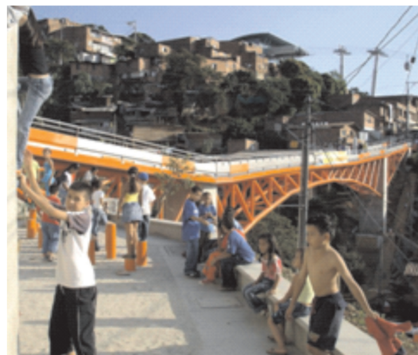
Figure 16. Andalucía Bridge - France.
