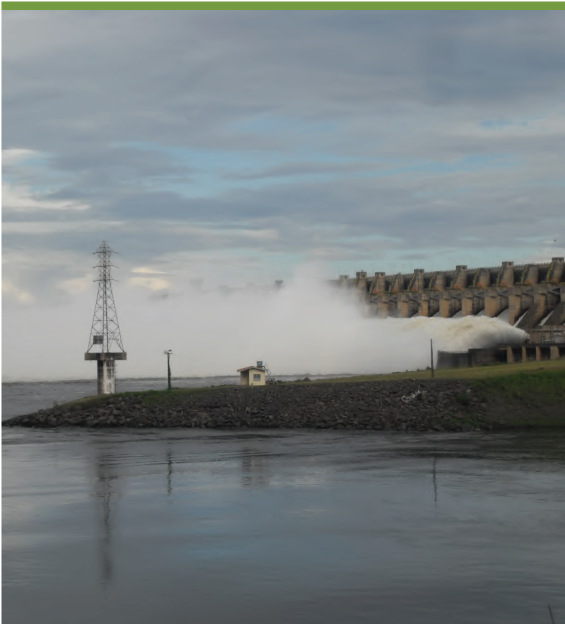
Tucuruí/PA Hydroelectric Plant. Photo: Diego Pereira
