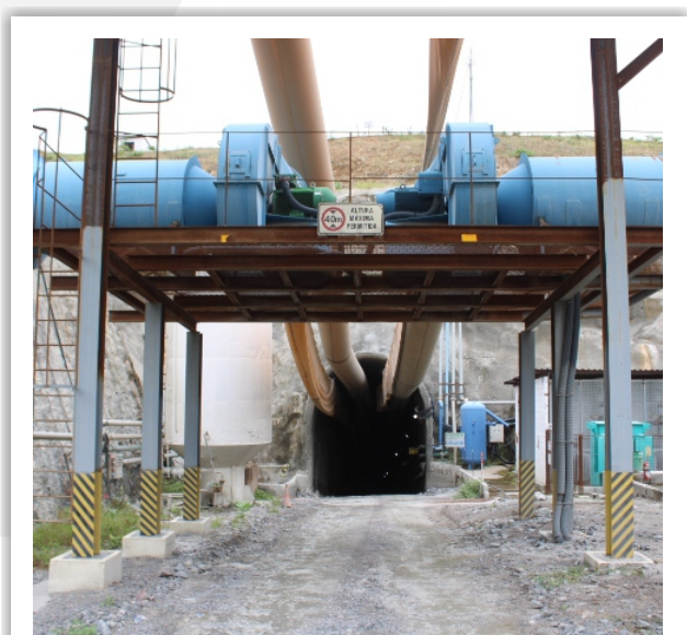
Janela do Túnel Major Sales.
