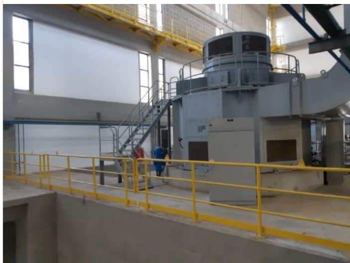
Figura 26-15 – EBI-2 – Cj. Moto-bomba instalado
