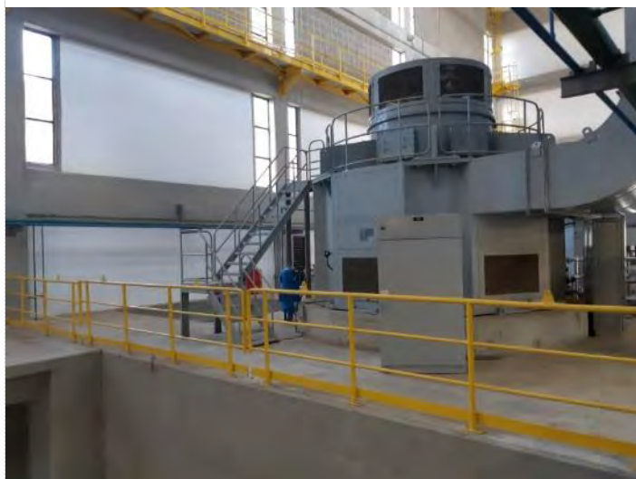
Figura 26-15 – EBI-2 – Cj. Moto-bomba instalado
