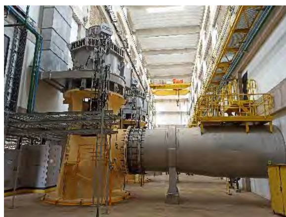
Figura 25-28 – EBI-1 – Bombas instaladas
