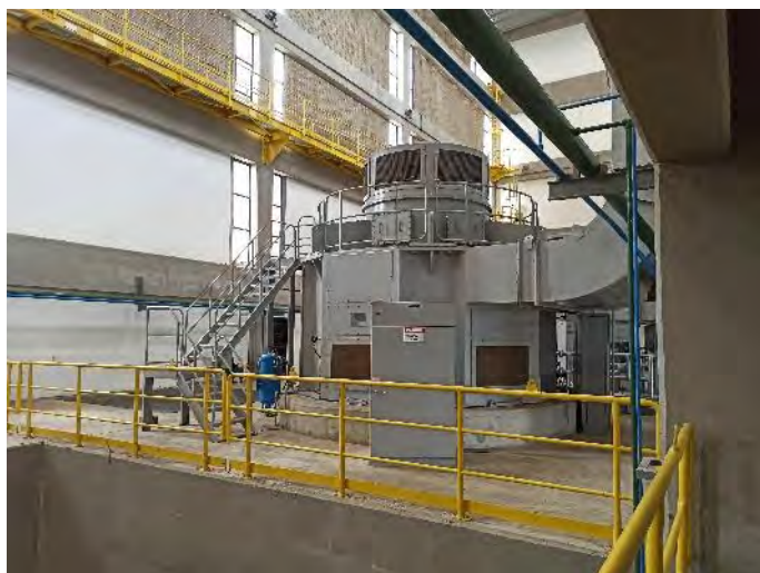
Figura 26-37 – EBI-2 – Cj. Moto-bomba instalado
