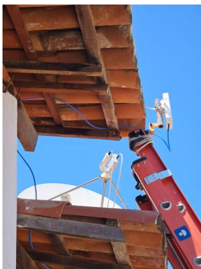
Figura 18 – ODU GX-5001 instalada.
