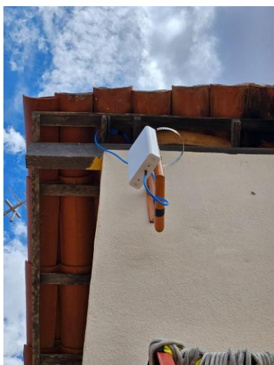
Figura 14 – ODU GX-5001 instalada.
