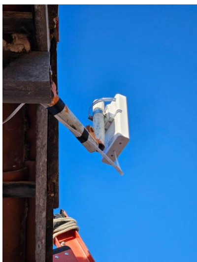
Figura 10 – ODU GX-5001 instalada.
