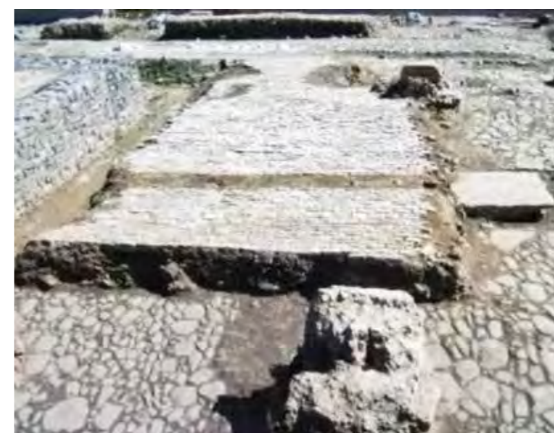
Figure 45. Section of paving stones from the Empress’s Wharf overlying the long section of slabs from Valongo Wharf.
