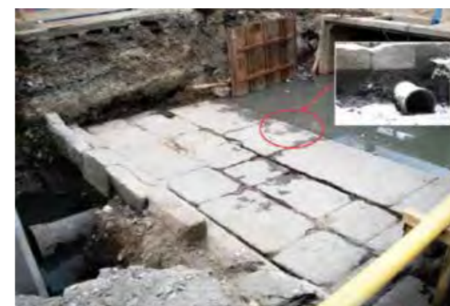
Photo 23 - Iron drainpipe under the structure. Source: Ibid., p.35
