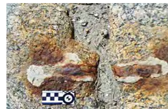
Photo 30 - stain around the remains of an iron clamp. Retrô archive. September 2014 – p.16
