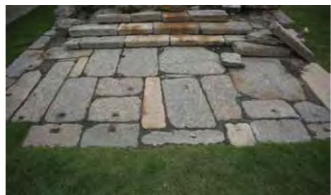
Photo 14 - Empress's Wharf. Cavities for clamps to attach the flagstones. Photo: João Maurício Bragança, 2014
