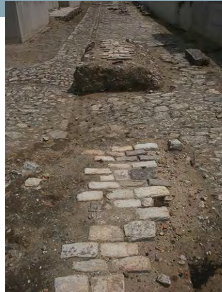
Figure 11. Paving of Valongo Wharf. Note at the centre of the photo the alignment of the cobblestones which function as the gutter for the drainage of rain water and, on the left, the lateral border of the wharf’s pavement, with flagstones carefully aligned. In the centre and to the left there are blocks pertaining to the paving of the Empress’s Wharf. Photo: João Mauricio Bragança, 2014.
