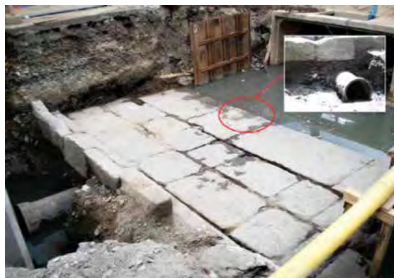
Figure 29: Iron drainpipe under the structure. Source: Ibid., p.35
