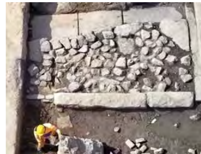
Photo 40 - Intervention made after the Empress's Wharf was built. Source: Ibid
