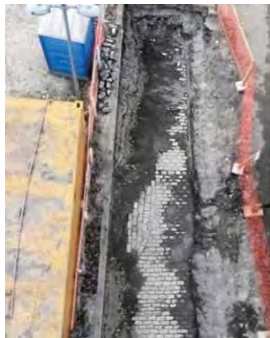
Photo 39 - Trench 17: section of parallel paving stones removed to make way for infrastructure developments in the area. Source: ANDRADE LIMA, Ibid., p.25
