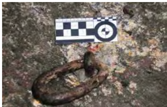
Photo 33 - Ferrous metal mooring ring displaying the way it was attached to the rock using lead. Source: ANDRADE LIMA, 2013
