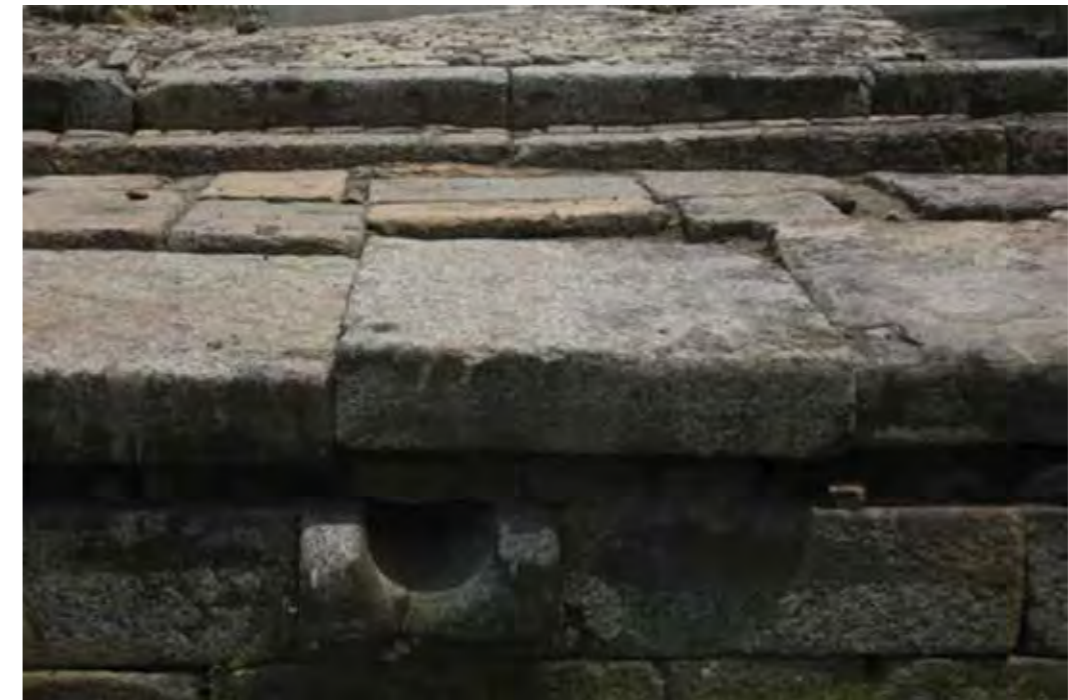
Figure 23. Empress's Wharf. Spout for draining off rain water. Photo: João Mauricio Bragança, December 2015.
