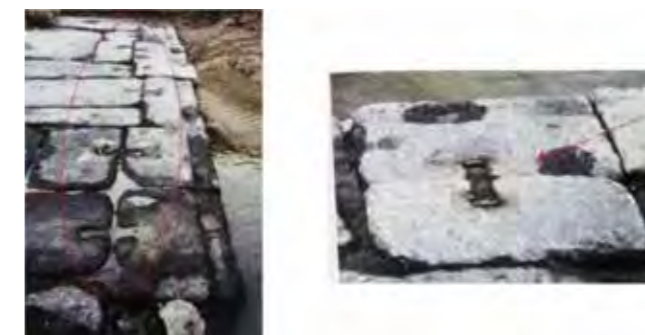
Photo 29 - Clamps or anchors used to fix the stones. Source: ANDRADE LIMA
