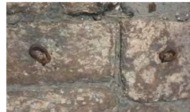
Photo 16 – Empress's Wharf. Detail of remnants of clamps to attach the flagstones. Photo: João Maurício Bragança, 2014
