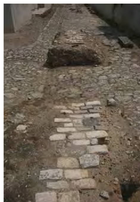
Photo 8 - Paving of Valongo Wharf. Note at the centre of the photo the alignment of the cobblestones which function as the gutter for the drainage of rain water and, on the left, the lateral border of the wharf's pavement, with flagstones carefully aligned. In the centre and to the left there are blocks pertaining to the paving of the Empress's Wharf. Photo: João Mauricio Bragança, 2014.
