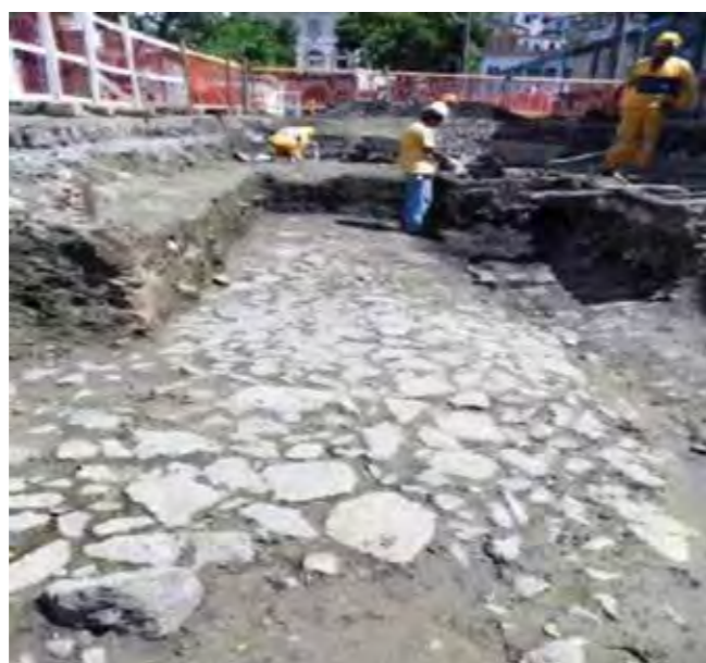
Photo 27 - South Section (left) and part of the West Section (right), divided by the Valongo Wharf gutter Source: Ibid., p. 44
