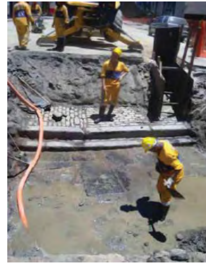
Figure 32. Flagstones, steps and parallel cobblestone paving revealed in front 2.
