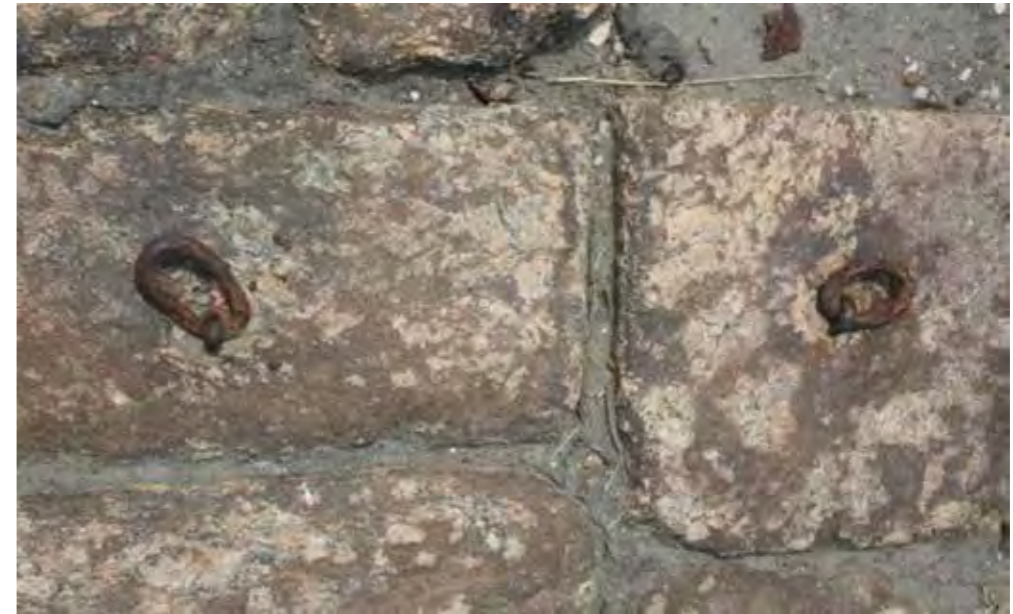
Figure 20. Empress's Wharf. Detail of remnants of clamps to attach the flagstones. Photo: João Maurício Bragança, 2014
