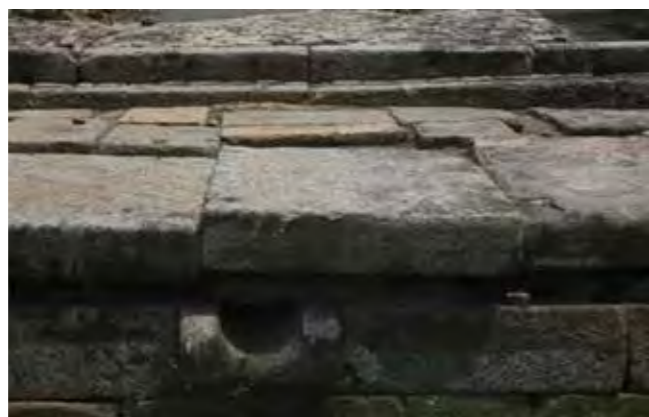
Photo 19 – Empress’s Wharf. Spout for draining off rain water. Photo: João Mauricio Bragança, 2014
