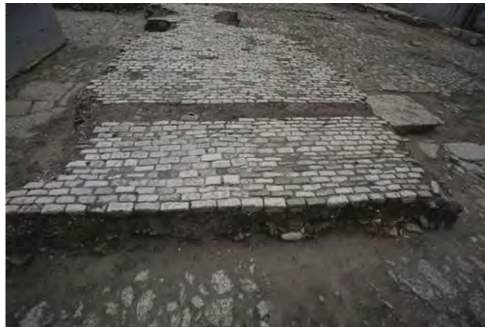
Figures 21 and 22 show fragments (demonstrative blocks) the Empress's Wharf with its regular cobblestone paving. Below it the pé de moleque paving of Valongo Wharf can be seen. Photos João Mauricio Bragança – November 2014 (top) and December 2015
