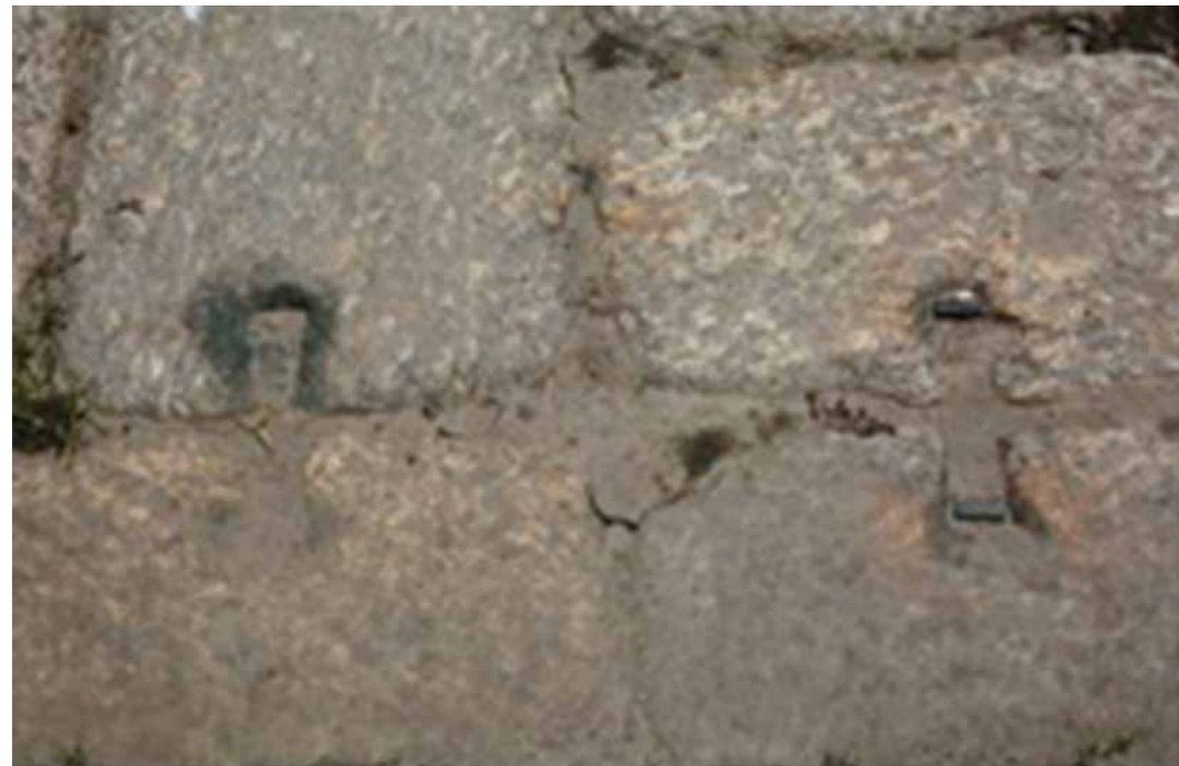
Figure 19. Empress's Wharf. Detail of remnants of clamps to attach the flagstones. Photo: João Maurício Bragança, December 2015
