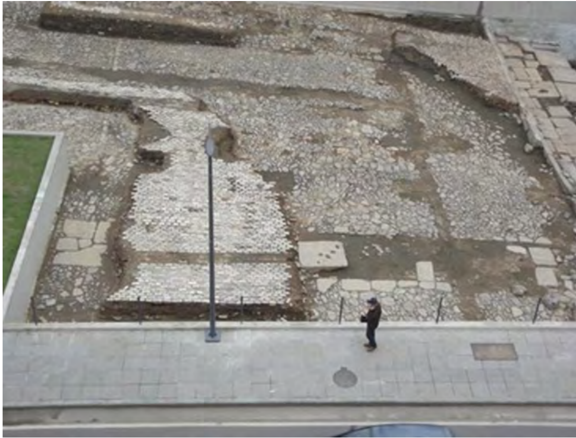
FIGURE 2 Pavement of the Valongo Wharf, made from uneven stones, deeper and better preserved. A few higher sections of pavement from the Empress Wharf survive, showing cobblestone bricks. Later trenches dug for the installation of underground utility networks are clearly visible. Photograph by authors.
