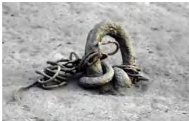
Photo 31 - Mooring ring embedded in the stone. Source: ANDRADE LIMA, 2013, p. 55
