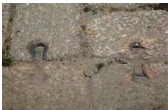
Photo 15 - Empress's Wharf. Detail of remnants of clamps to attach the flagstones. Photo: João Maurício Bragança, December 2015
