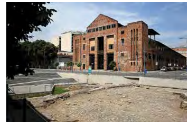
Photo 76 - View of the main facade of the Docas D. Pedro II building. In the foreground, remains of Valongo and Empress Wharves. Photo:João Maurício Bragança, December 2015
