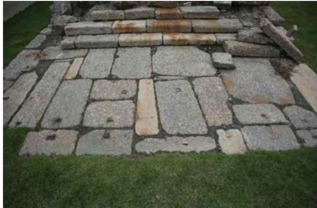
Figure 18. Empress's Wharf. Cavities for clamps to attach the flagstones. Photo: João Maurício Bragança, 2014
