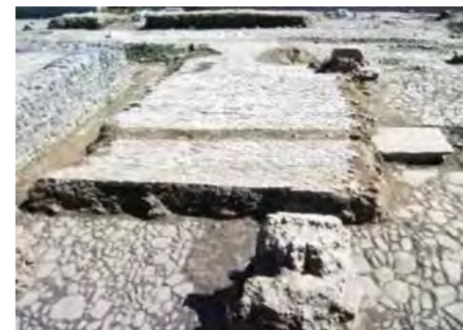
Photo 36 - Section of paving stones from the Empress's Wharf overlying the long section of slabs from Valongo Wharf Source: ANDRADE LIMA, 2013, p. 55
