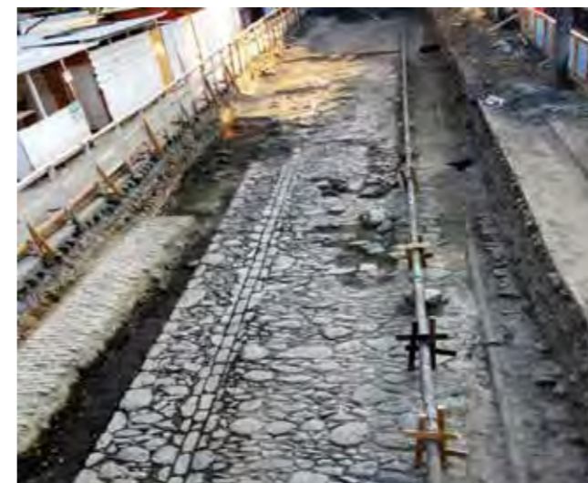
Photo 42 - Front 4 – paving stones indicating the existence of a gutter. Source: Ibid., p. 69
