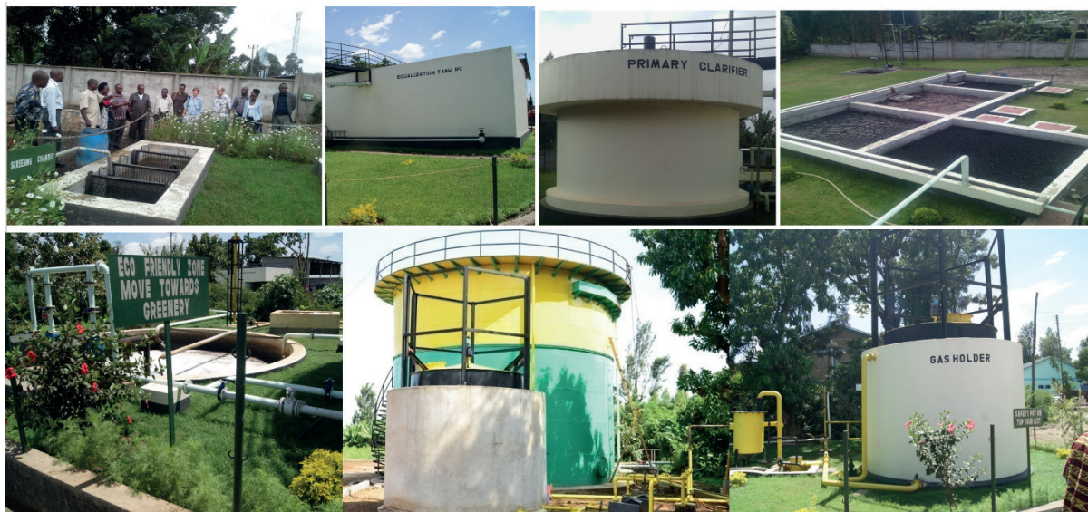
Figure 10. Facilities installed to meet the objectives of adequately treating banana wine wastewater, a. recovering nutrients and producing biogas, b. recovering water for re-use and c. beautification. From left to right: (1) Screening (2) Equalization (3) Clarification to produce sludge (3) Sludge dewatering for reuse (4) Buffer tank (5) Biodigester (6) Biogas holding. Observe the whole beautification of the treatment area.
