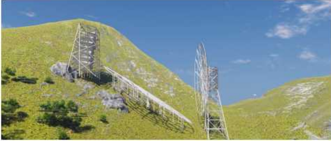
Figure 3.1 - The artistic view of the BINGO telescope site. This figure displays the sheltering hill and the use of the natural inclination of the terrain to place the primary and secondary mirrors, in addition to the horn structure.
