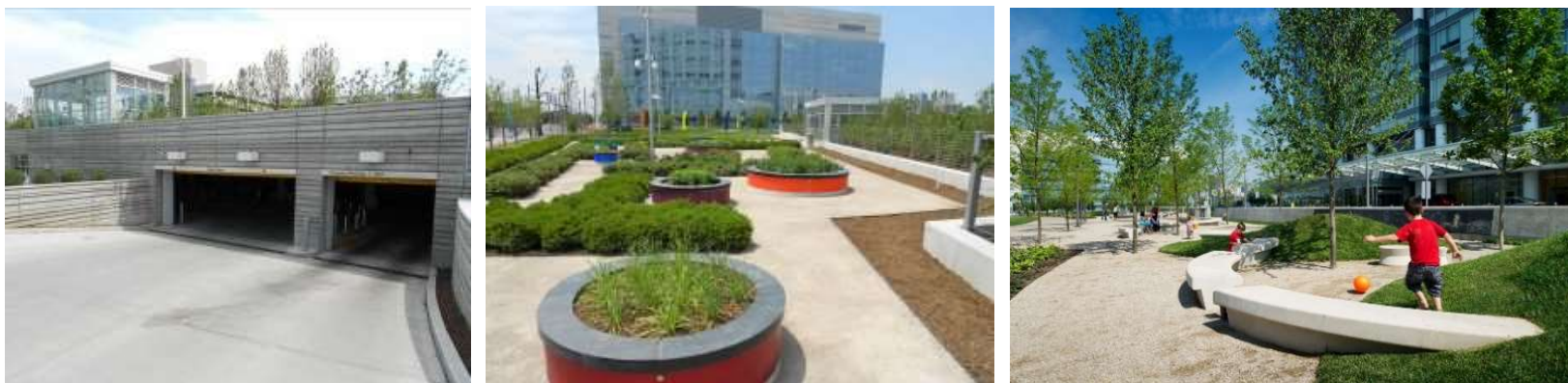
Figura 43: Nationwide Children's Hospital da Faculdade de Medicina da Universidade Estadual de Ohio (fonte: https://walkerconsultants.com/projects/nationwide-childrens-hospital-underground-garage ).
