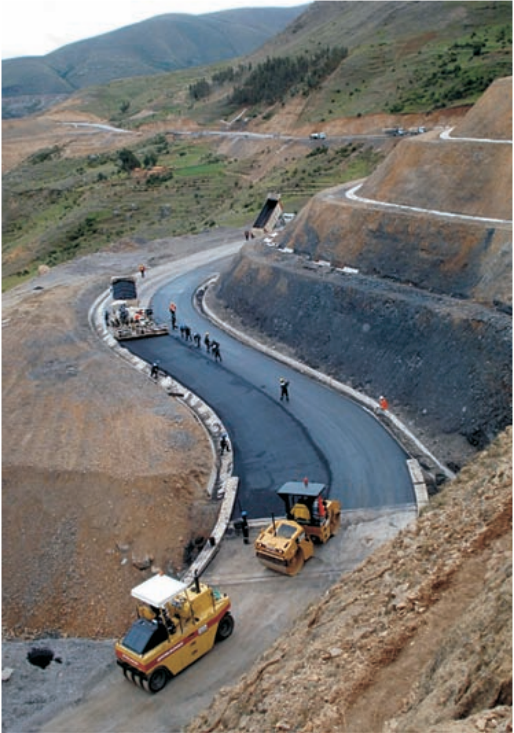
Workmanships in execution in the South Iirsa, Stretch 2, in Peru
