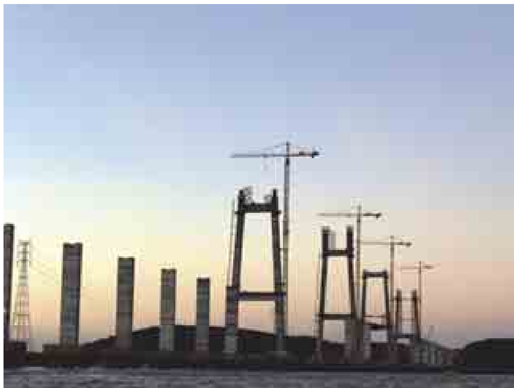
Roadway System and Rail-and-Road Bridge spanning the Orinoco River
