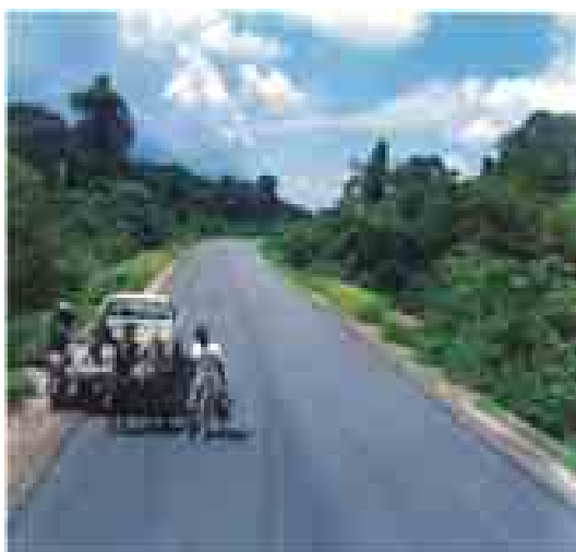
Road concluded: built by Andrade at Congo
