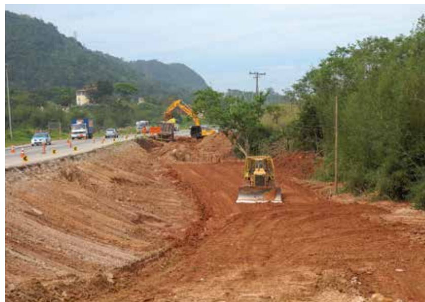
BR-101/RJ - Trecho Santa Cruz-Mangaratiba
