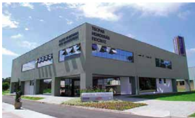
IBMP plant for the production of the reagents to be developed by the INCT studies
