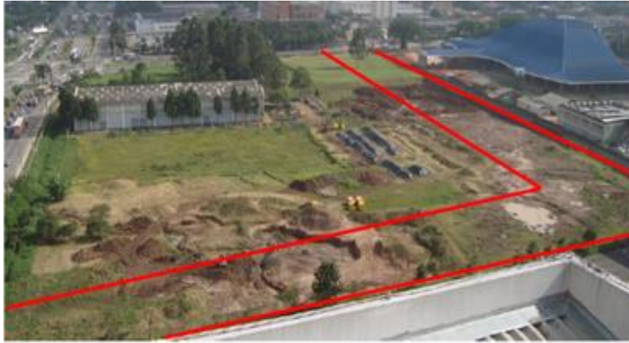
Figure F.7 - UDSP - the red range represents the decontaminated area - 18,400 m 2
