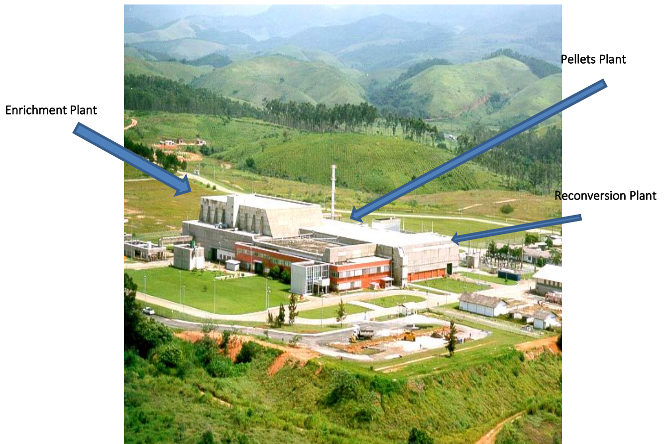
Figure 4 – The Unit of Enrichment, Reconversion and Fuel Pellets Facilities - Resende/RJ
