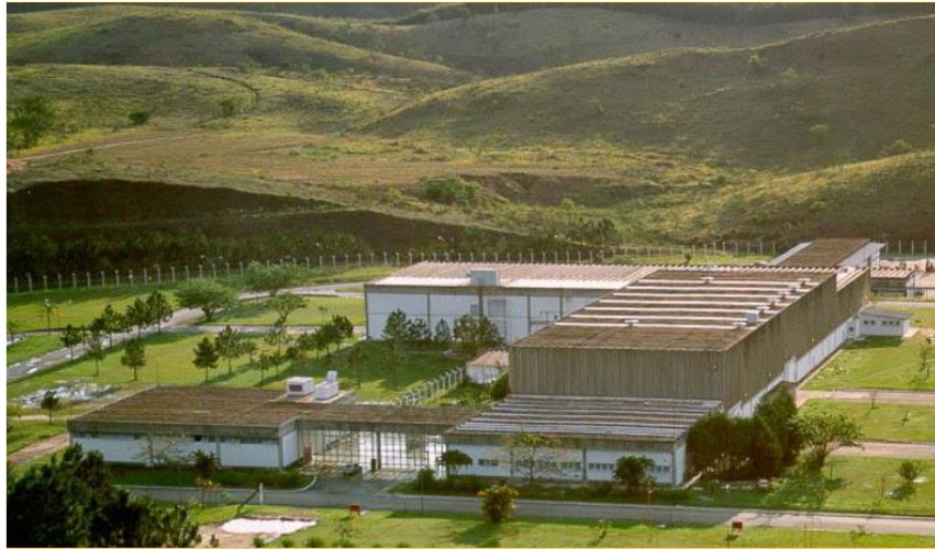
Figure 5 – The Unit of Fuel Assembly – Resende/RJ
