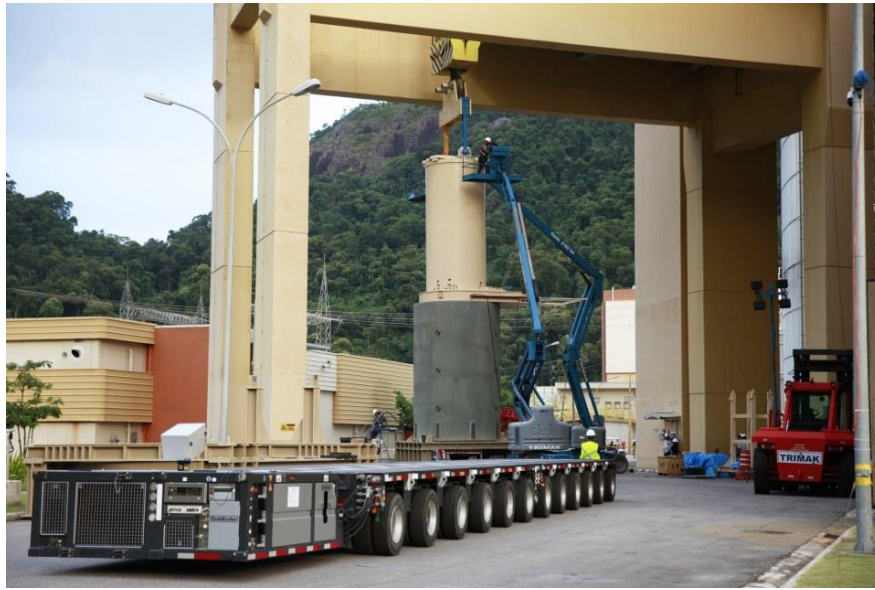
Figure 24 - Canister transfer from Hi-Trac to Hi-Storm (Credit: ABDAN)
