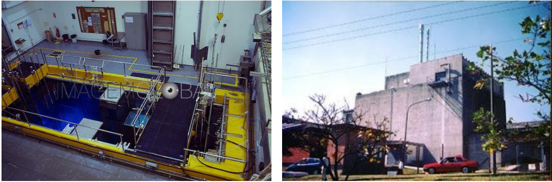
Figure 6 - IEA-R1 – Pool of Reactor and Reactor Building
