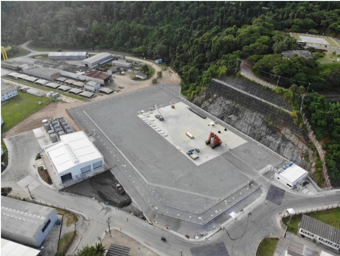
Figure 26 - Aerial photo of UAS during movement of the first HI-Storm (Credit: ABDAN)
