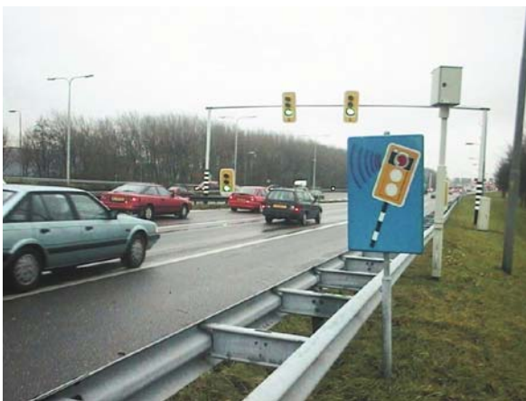
Freeway Traffic Management and Control, Figure 7 Ramp metering at the freeway A13 in Delft, The Netherlands. One car may pass per green phase. To prevent red-light running the control is enforced
