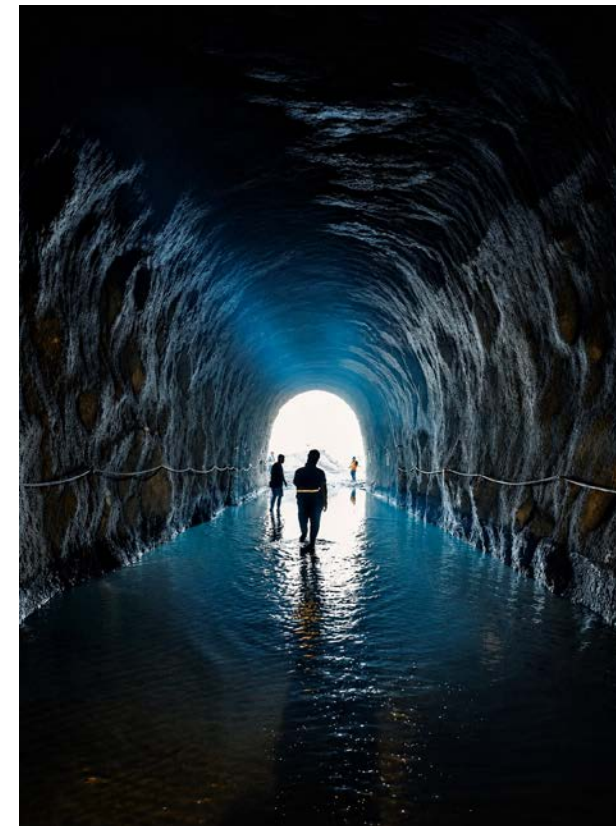
Túnel Major Sales Ramal do Apodi/RN
