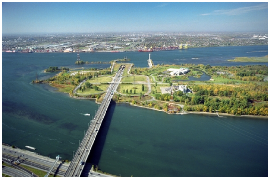
Figura 15: ponte-túnel Louis-Hippolyte-LaFontaine , Montreal
