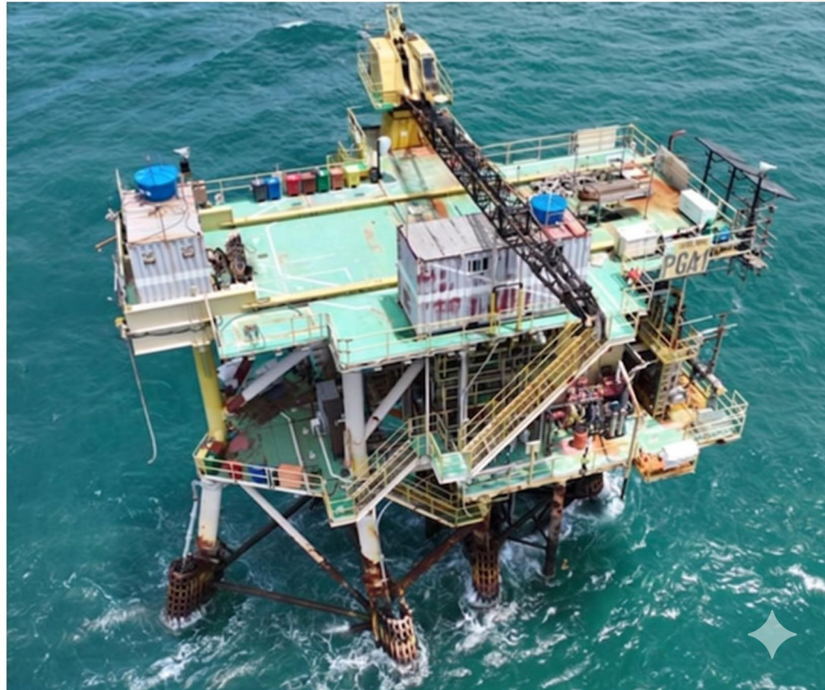
PGA-1 at its location (September 2022)
