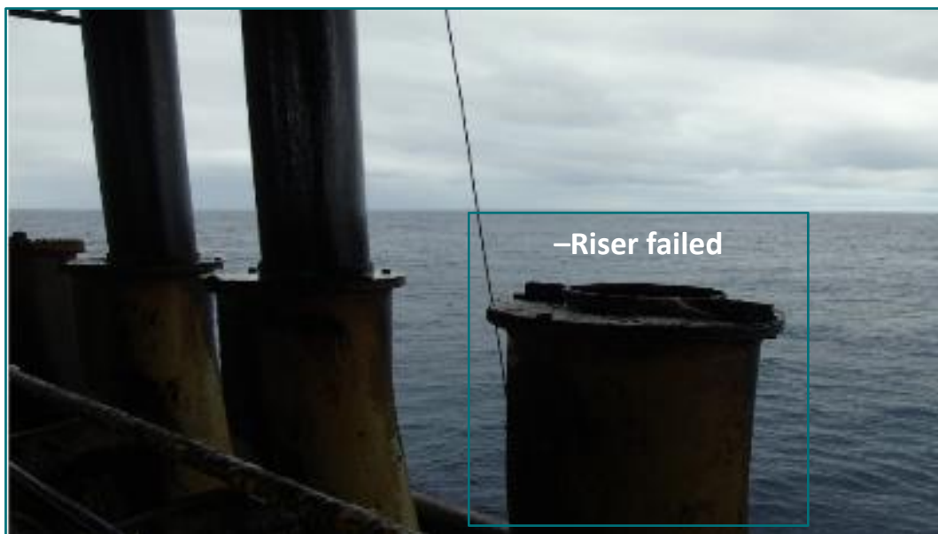
Figure 1 - Location of the I-tube of the ruptured riser (spider deck)
