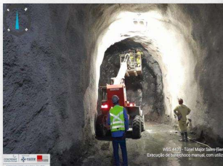
Túnel Major Sales Janela sentido Emboque
