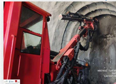
Túnel Major Sales Emboque
